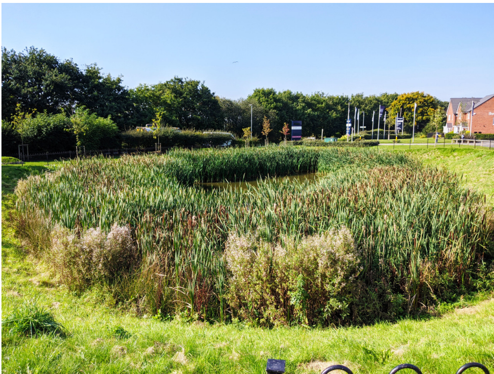
Picture 3.2 Sustainable drainage solutions such as this pond and reed bed reduce flood risk whilst also enhancing biodiversity and improving water quality.
