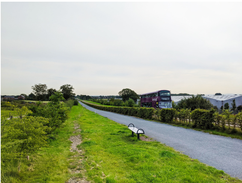
Picture 3.5 The Leigh Salford Manchester Guided Busway has a 3m multi user route running its length through the borough and has been highly successful in encouraging walking and cycling.
