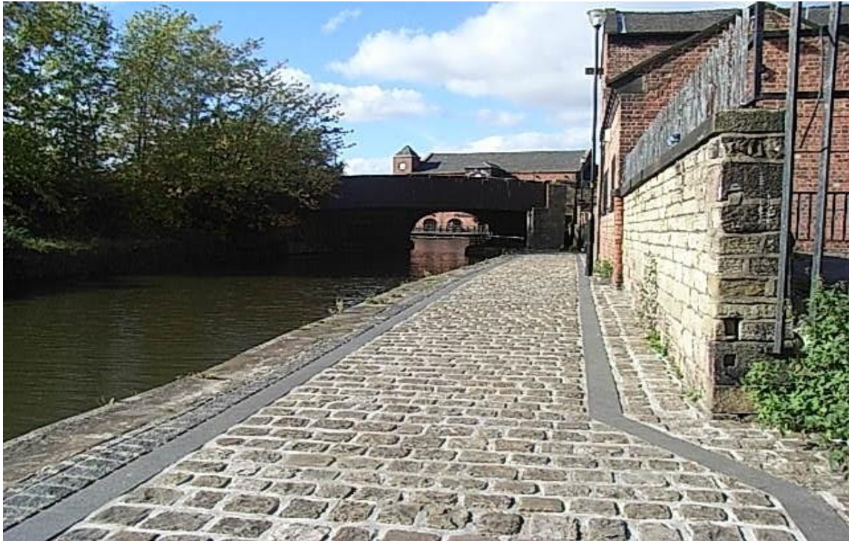
Figure 2 Towpath improvements at Wigan Pier
