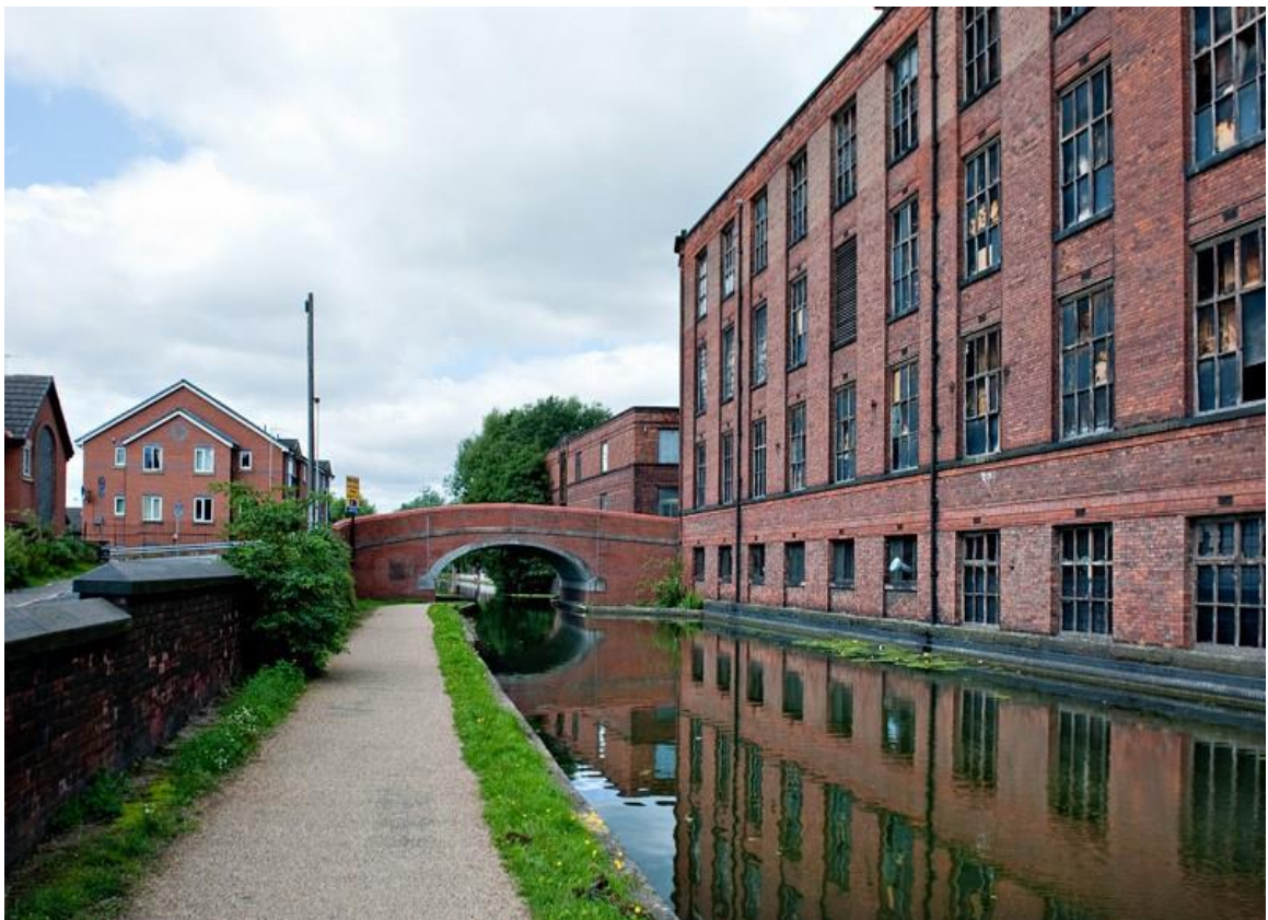
Figure 4 Mather Mill, Leigh under restoration
