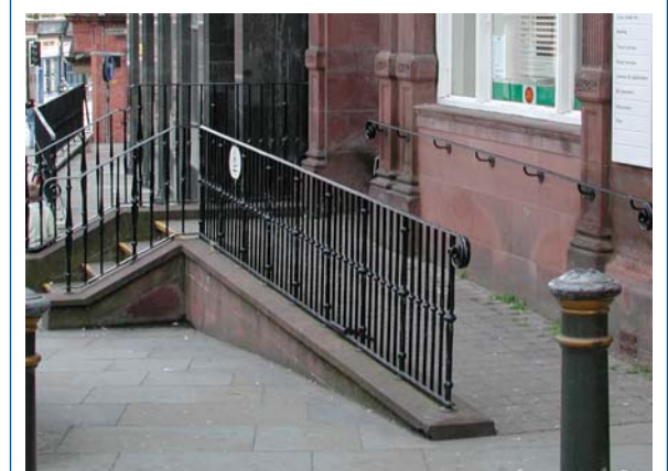
Good example of a ramped access with associated steps
