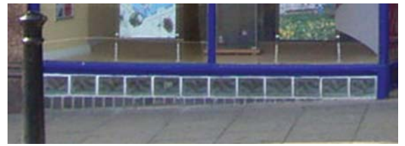
Example of glass blocks stallriser. This material has been used to help natural light filter through to the basement
