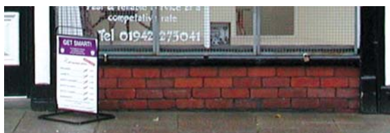
Example of a brick stallriser
