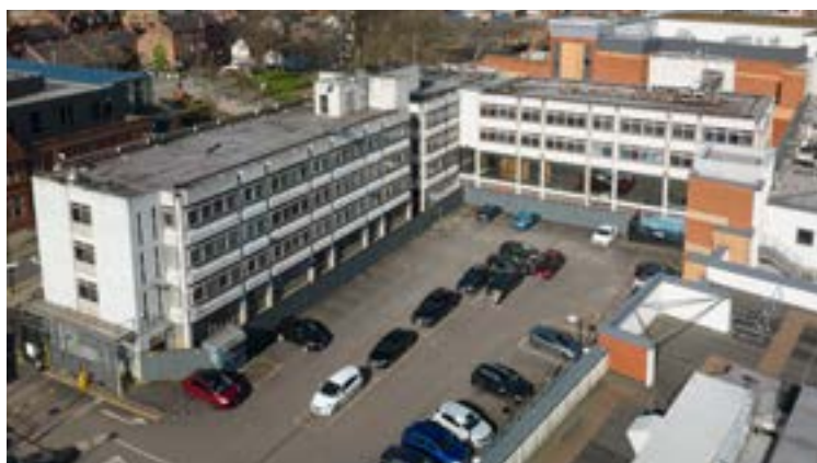
An aerial view of the Civic Centre
