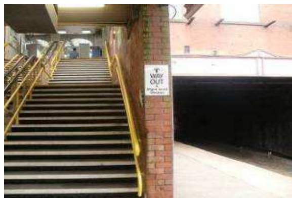
Photo 2.12: Platform Steps and North Western Sign
