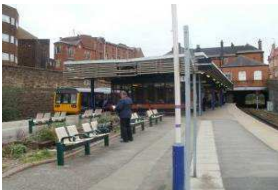
Photo 2.11: Platform 1 and 2 Waiting Facilities
