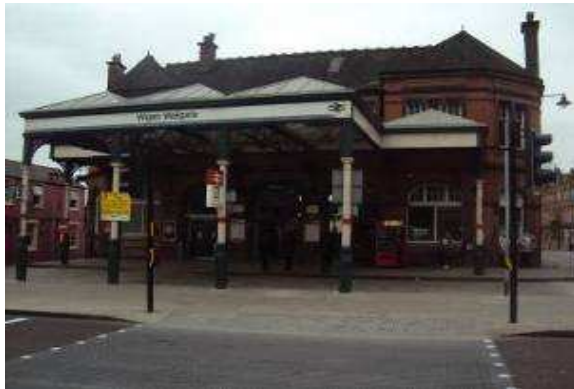
Photo 2.7: Wigan Wallgate Railway Station Canopy
