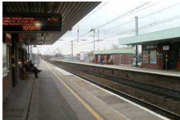
Photo 2.6: North Western Platforms
