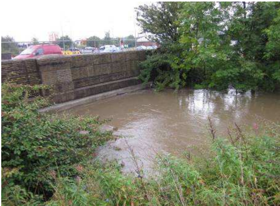
Figure 6: Adam Bridge - River Levels up to Soffit Level Preventing Discharge
