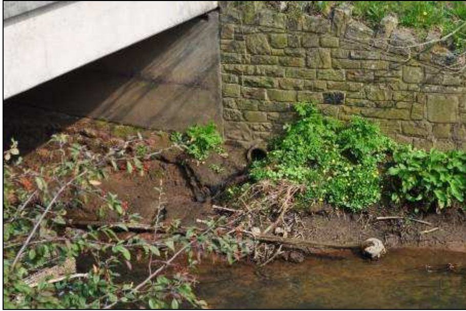
Figure 5: Existing Surface Water / Highway Drainage Outfall – Normal Conditions
