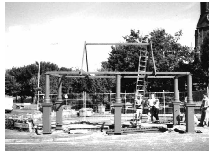
Well Sections made and installed by Tom Price's 'Camba' Works
