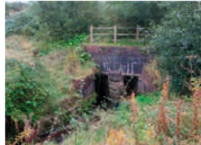
Honksford Brook passing through culvert beneath Guided Busway
