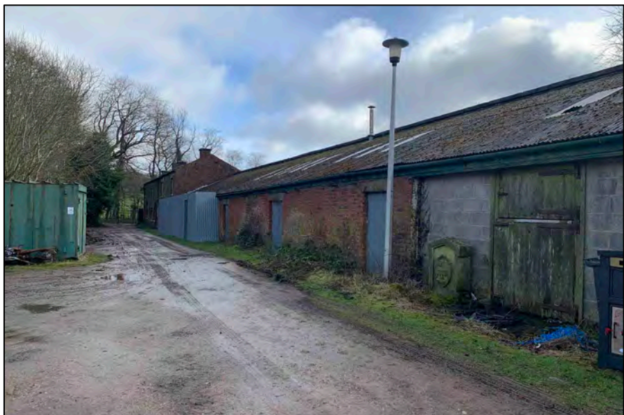
Appendix 2.3: View of front elevation of Bothy Range looking East
