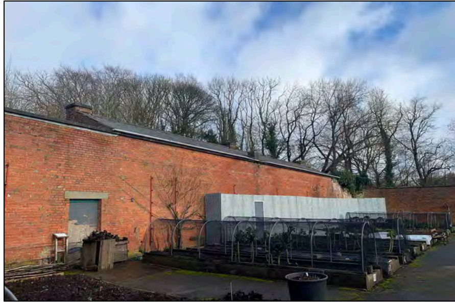
Appendix 2.4: View of rear elevation of Bothy Range looking East
