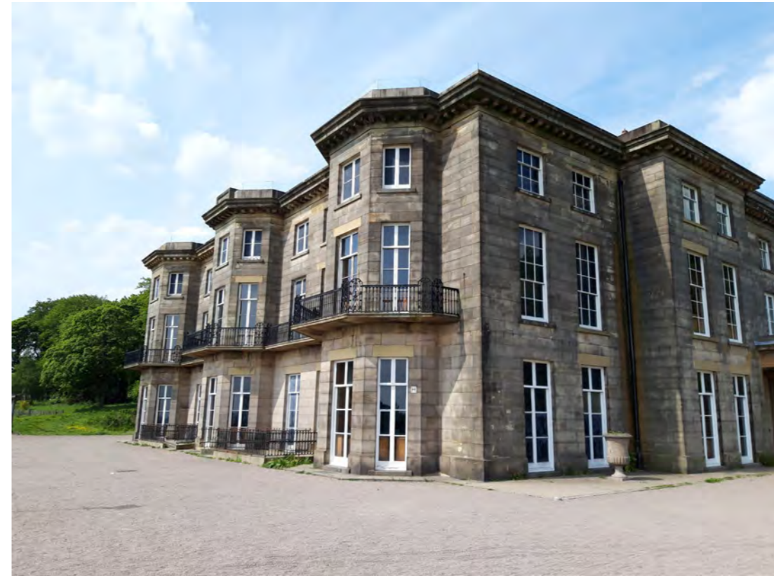
The south-east / south west elevations
