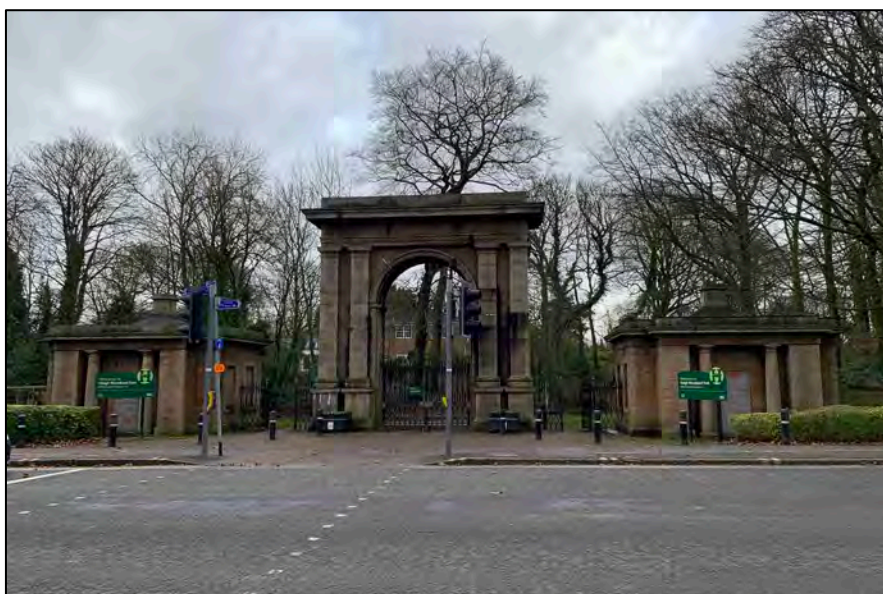
Appendix 2.11: View of Plantation Gates (listed at Grade II* NHLE: 1284570) looking East
