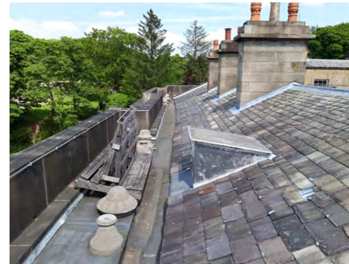
The loose urns on the roof with the potential for reinstatement
