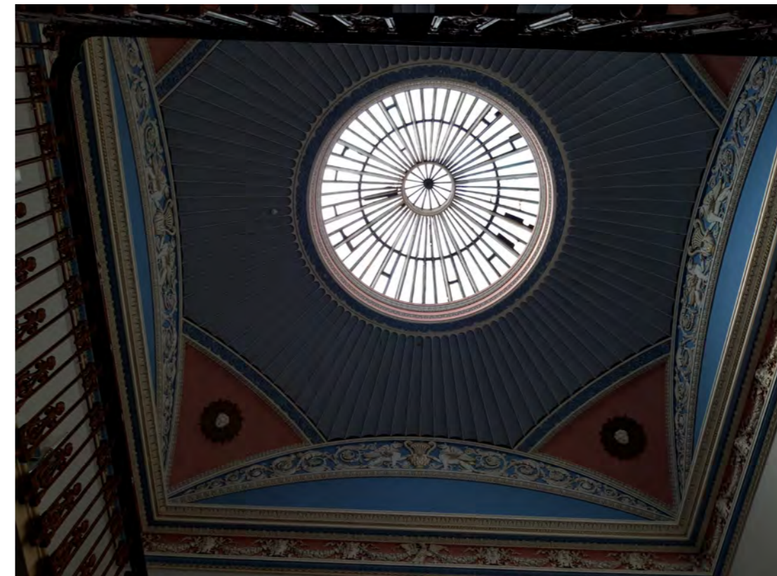
The sail vault over the Grand Staircase
