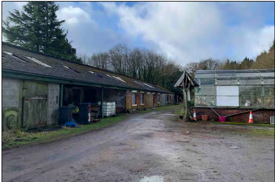
Appendix 2.2: View of western part of front elevation of Bothy Range looking West
