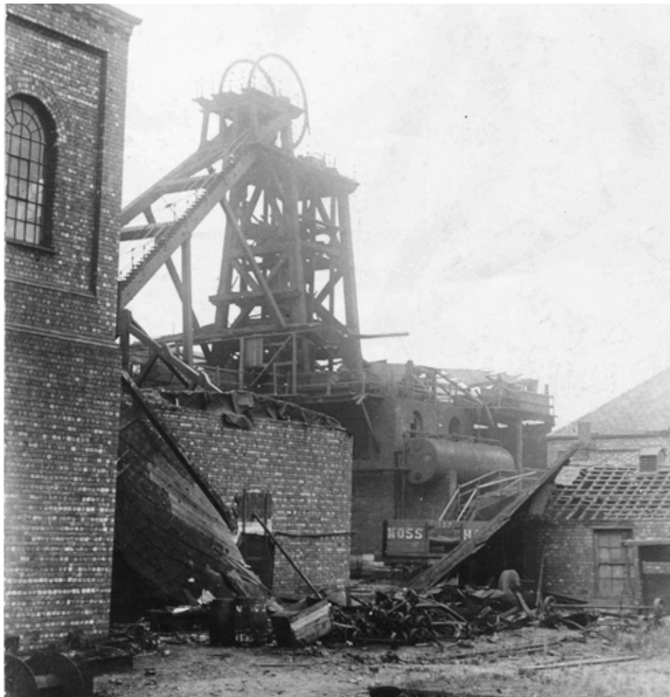
Damage to shaft at Maypole Colliery 18 August 1908
