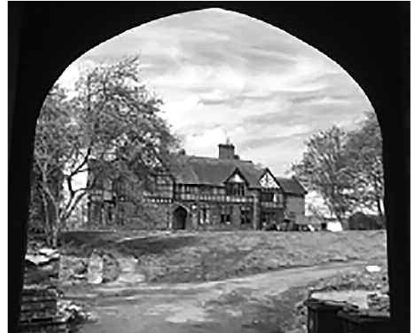
Work on the Hall underway, taken from the Gatehouse
