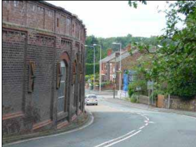
Image 12: Former bleach works wall, Chorley Road
