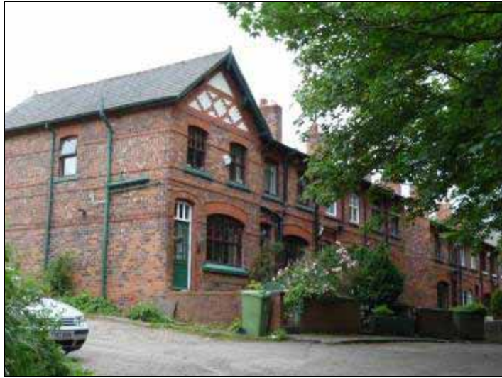
Image 49: Replacement windows on Mayflower Cottages
