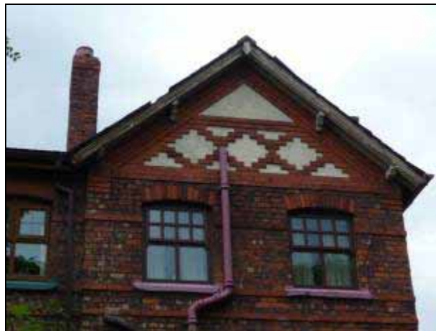
Image 42: Brick detailing on front gables to Mayflower Cottages
