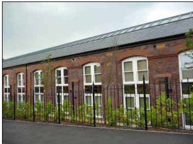
Image 37: Former Engine House
