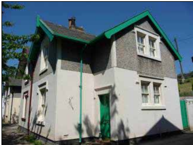
Image 29: Architectural details at Lakeside Cottages
