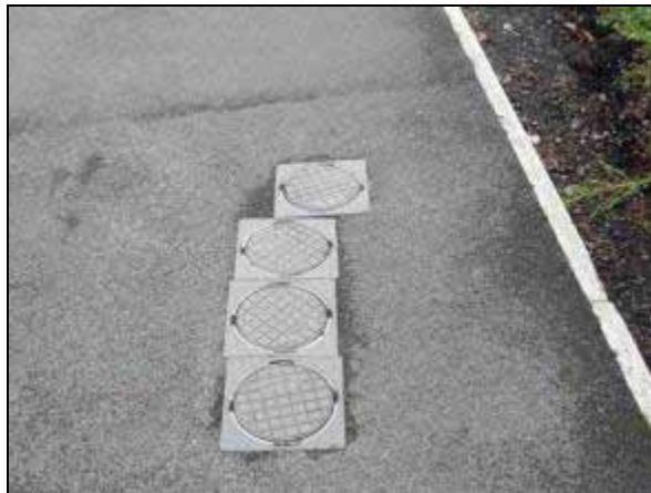
Image 48: Raised drain covers on pavement
