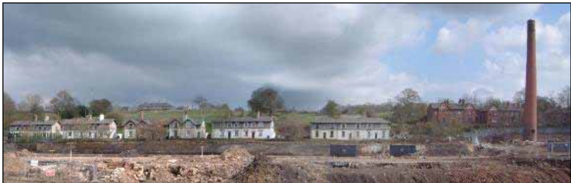
Image 34: View of Lakeside Cottages during demolition of the bleach works
