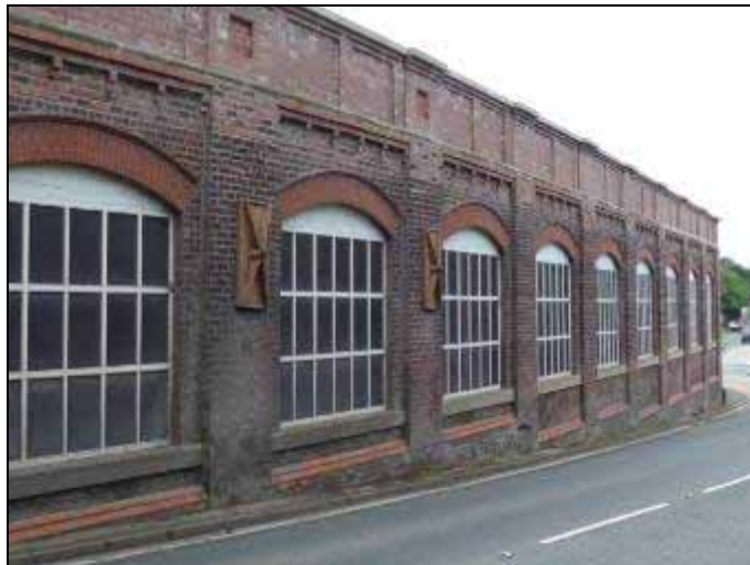
Image 13: Former bleach works wall, Chorley Road
