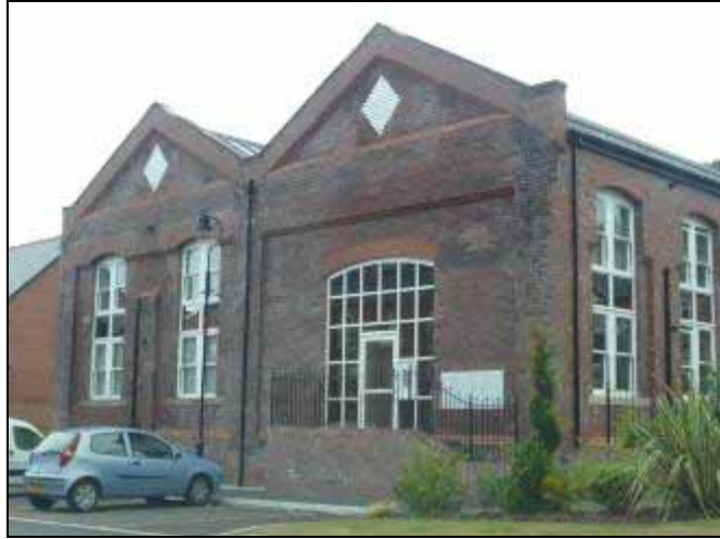
Image 38: Former Engine House: Front Elevation
