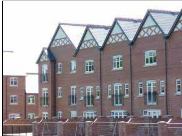
Image 44: Brick detailing to rear gables on new development
