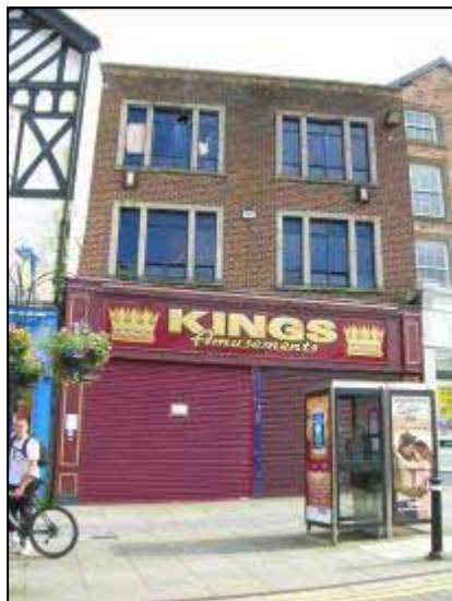
Photograph 49: example of unsympathetic shop front
