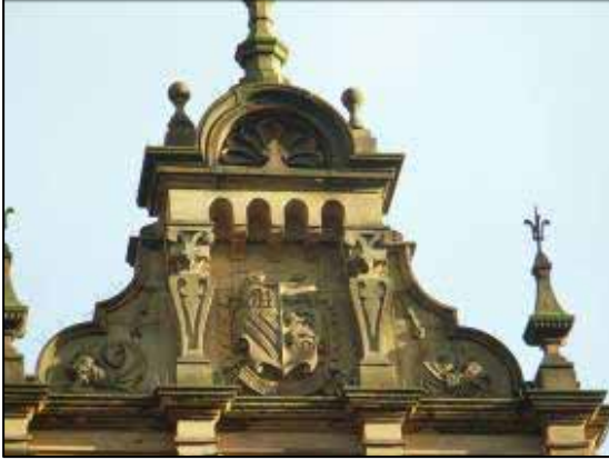
Photograph 39: Stone detailing on roof
