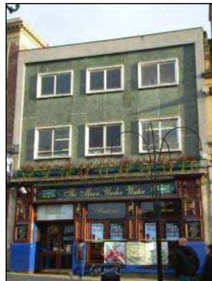
Photograph 40: example of unsympathetic infill development
