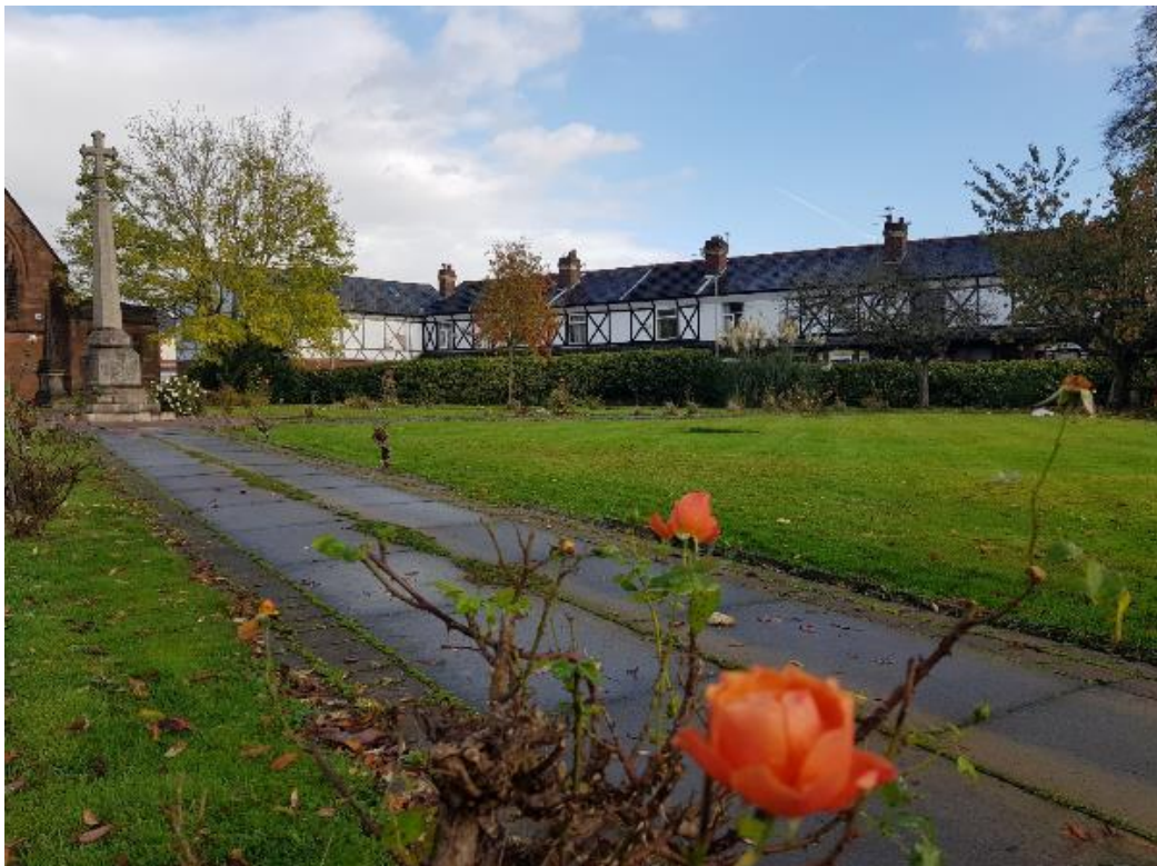
Picture 29. The late 19 th century Church Terrace overlooking St Thomas Church.
