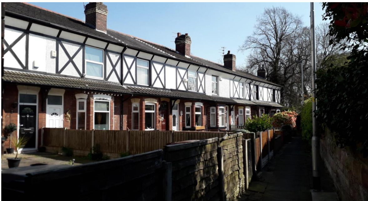
Picture 38. Church Terrace showing details of timber cladding and chimneys.
