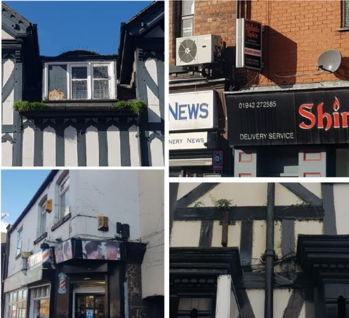
Picture 25 Clutter and poor repair is evidenced in the conservation area.
