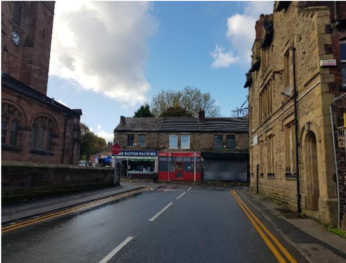
Picture 20. Local sandstone facing the buildings at Heath Road
