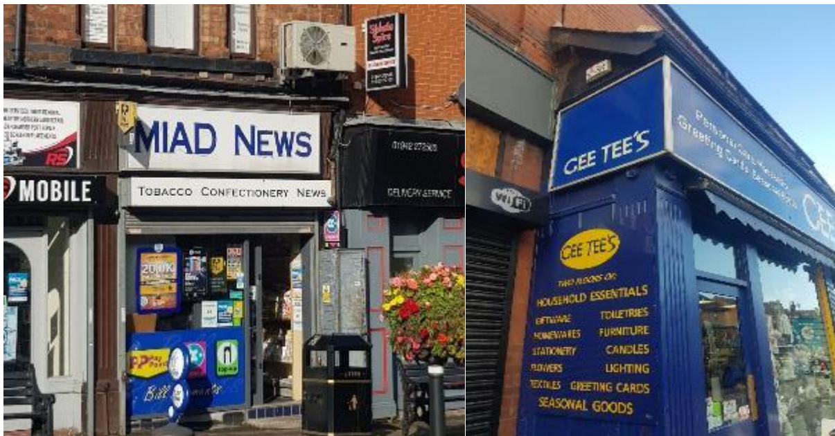
Picture 24. Poor quality shopfronts including dominant and unattractive signage, clutter and inappropriate attachments.
