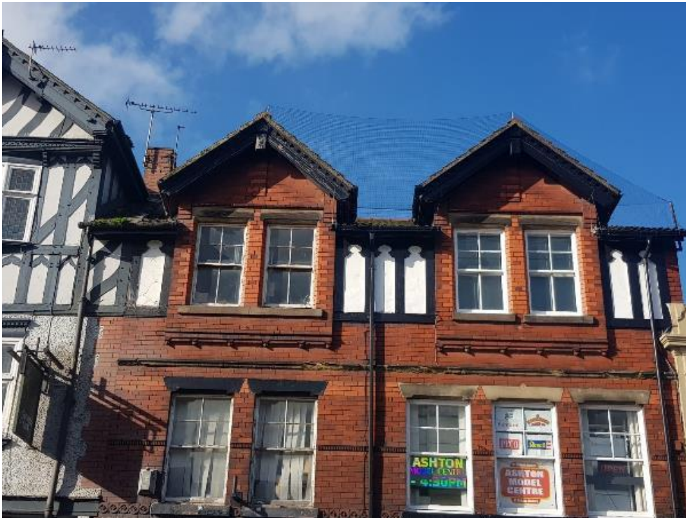
Picture 12. The area is typified by strong front-facing gables and gabled dormers.
