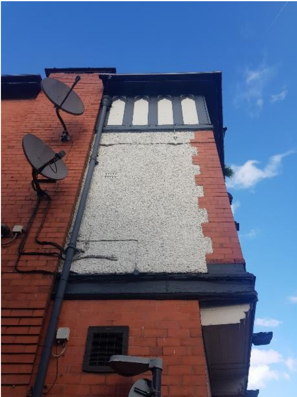
Picture 19. Brick, pebble-dash and mock-timbering are common materials in this character area, often on the same building.
