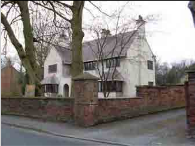
Photo 8: Detached residence, Church Road
