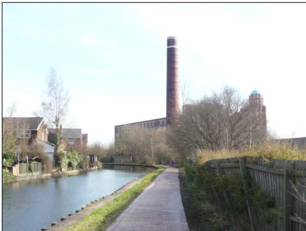
Photo 58: View of Butts Mill eastwards
