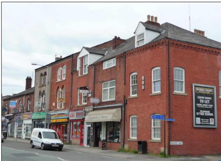
Photo 4: Chapel Street, Leigh
