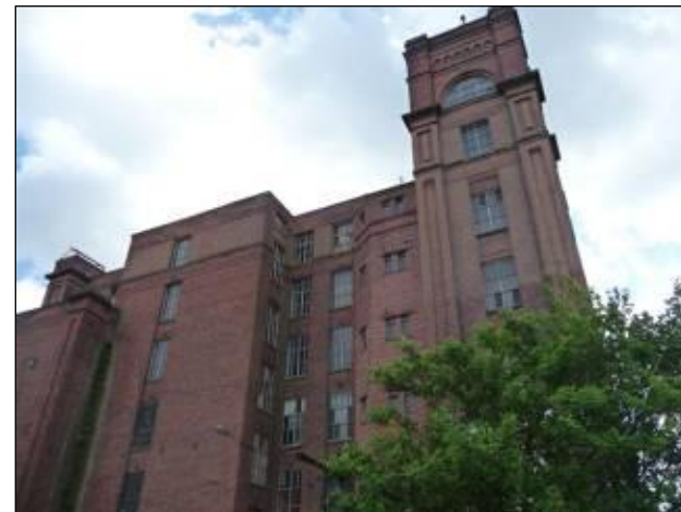
Photo 31: Side elevation of Mather Lane Mill
