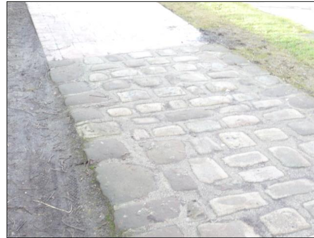
Photo 64: Cobbled stone surfacing along the Bridgewater Canal Towpath
