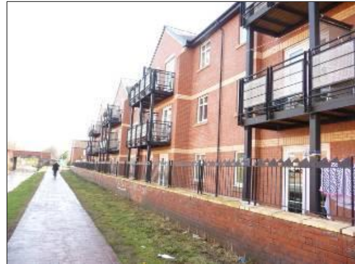
Photo 23: New housing along the Bridgewater Canal
