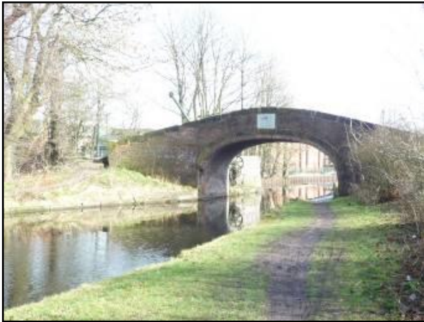
Photo 48: Hall House Bridge
