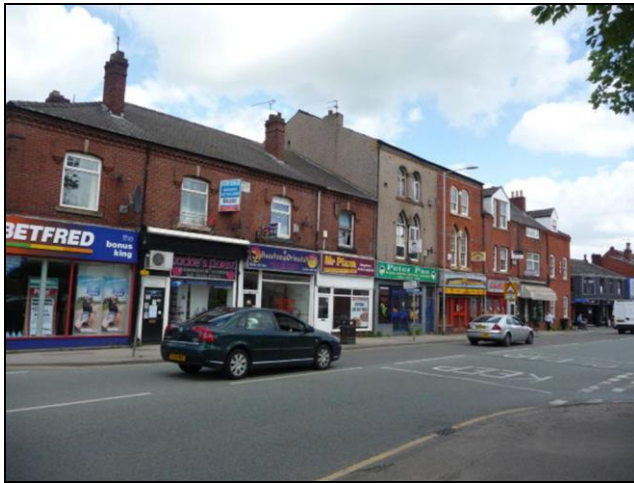
Photo 6: Chapel Street frontages
