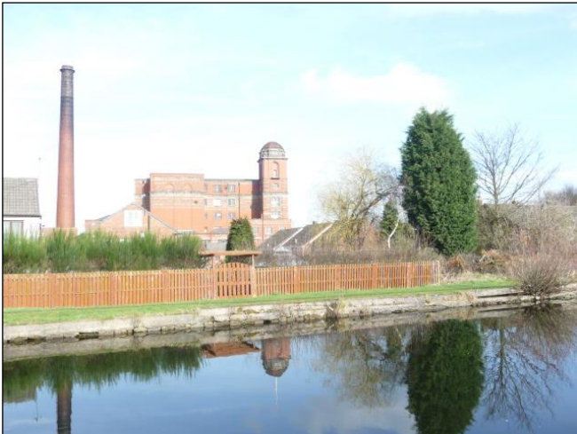
Photo 55: Leigh Spinners is a key landmark building in the Bridgewater Canal Conservation Area
