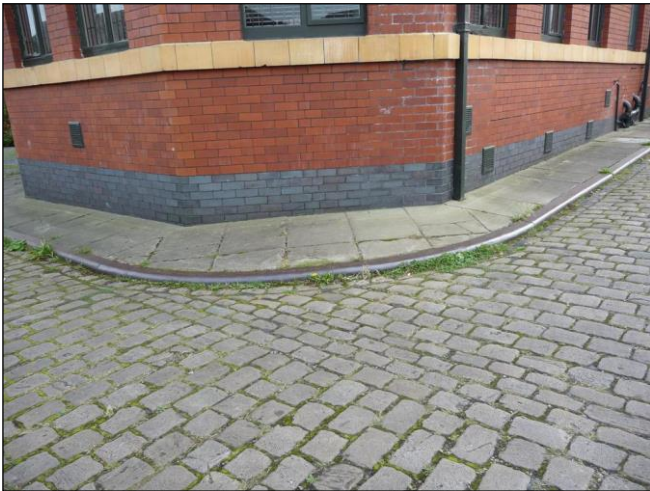
Photo 66: Cobbled surface at Alder Mill offices
