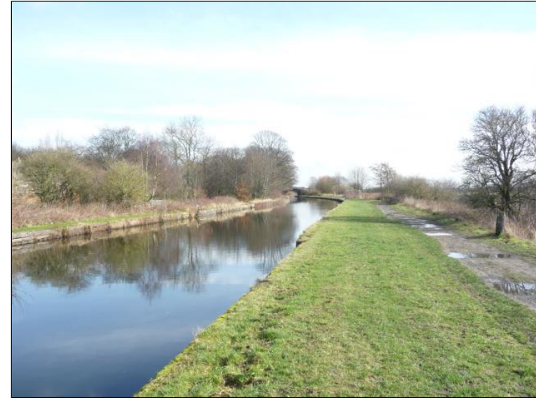
Photo 62: View eastwards towards Hall House Bridge
