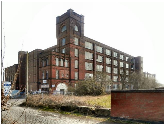
Photo 63: Remnants of original cobbled surfacing to the foreground of Brooklands Mill
