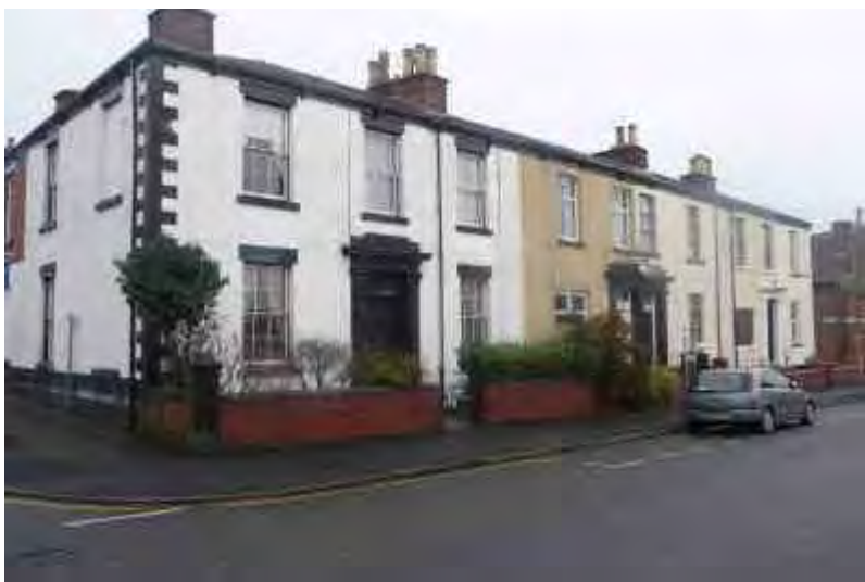
Figure 43 - 4 Lansdowne Terrace, Earl Street
