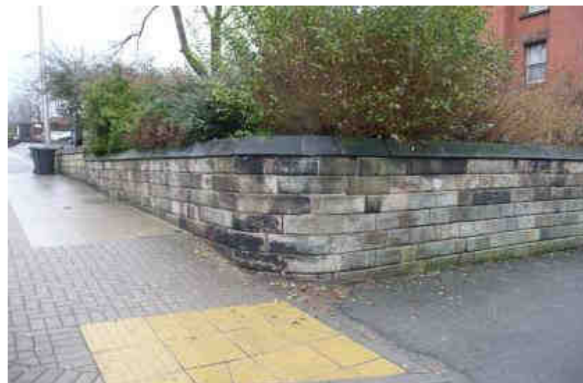
Figure 23 - Stone boundary wall and path outside St Mary's Presbytery, Standishgate.
