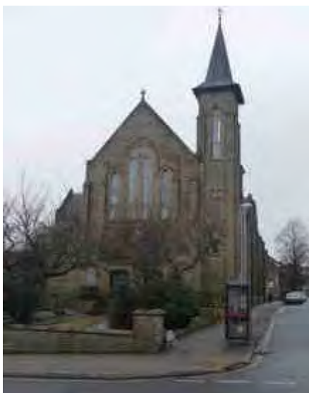
Figure 28 – Former St Paul's Congregational Church
