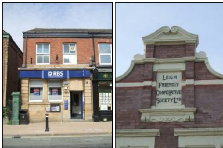
Photograph 11 (left): Stone at ground level of 68 High Street. Photograph 12 (far left): Stone detailing at roof level.
