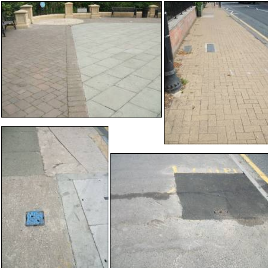
Photographs 20-3: Examples of good and bad paving surfacing within the conservation area.
