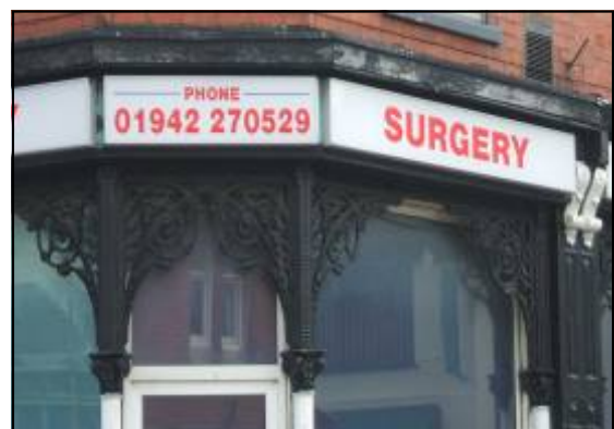
Photograph 30: Historic details on 107-109 High Street
