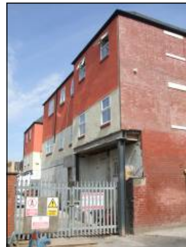
Photograph 32: Rear development at 26 Heath Street
