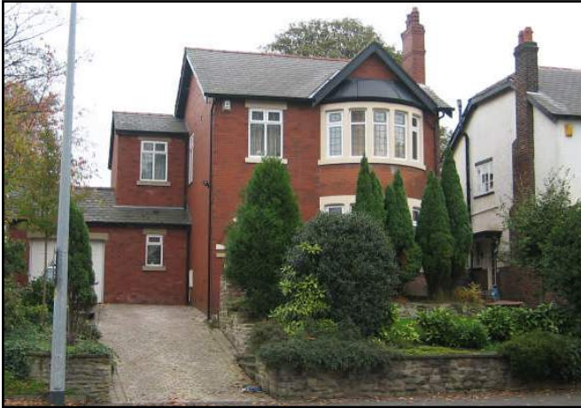
Photograph 75A: 323 Wigan Lane (Viewed From Wigan Lane)
