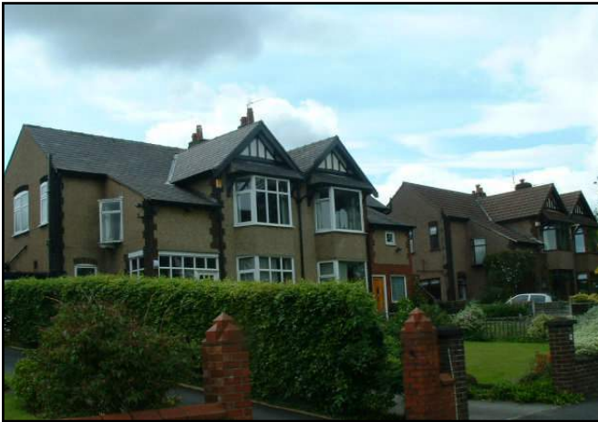
Photograph 107: 30 & 32 Brock Mill Lane (Viewed From Brock Mill Lane)
