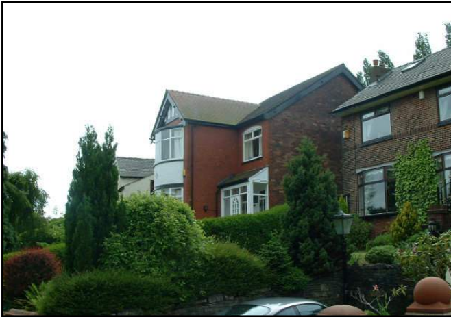
Photograph 104A: 18 & 20 Brock Mill Lane (Viewed From Brock Mill Lane)
