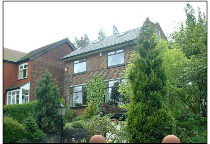
Photograph 104B: 18 & 20 Brock Mill Lane (Viewed From Brock Mill Lane)
