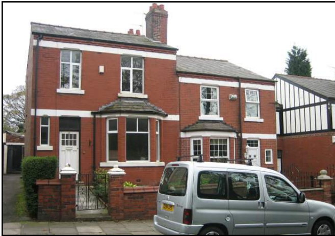
Photograph 24: 6 & 8 Walter Scott Avenue (Viewed From Walter Scott Avenue)
