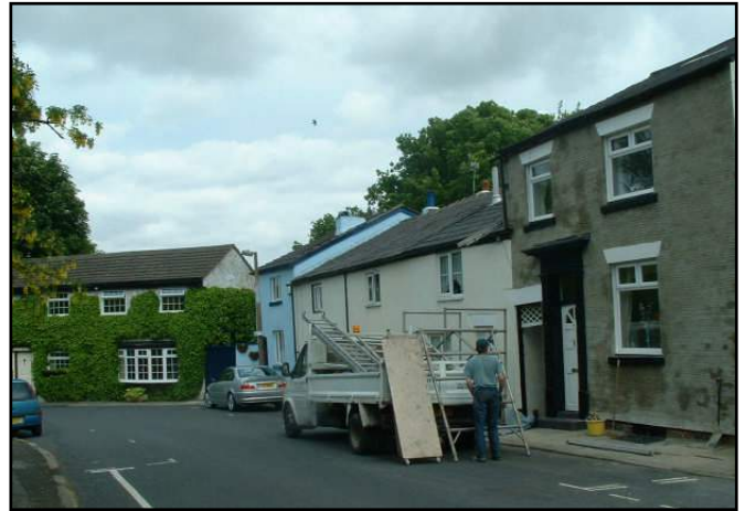
Photograph 110: 3 Brock Mill Lane (Viewed From Brock Mill Lane)
