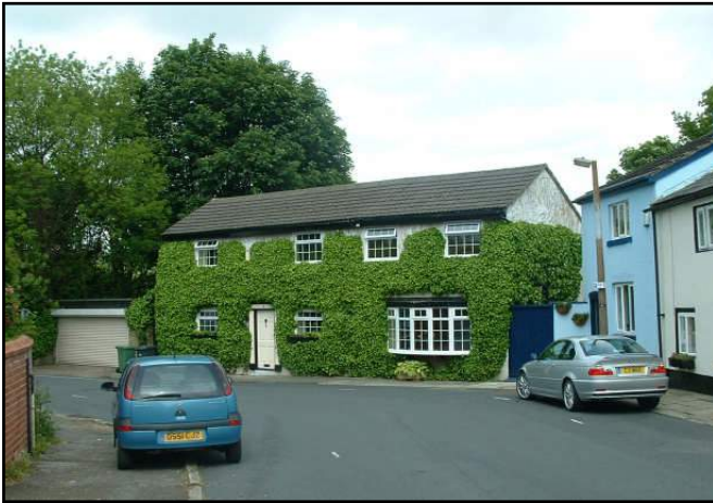
Photograph 109: 5 & 9 Brock Mill Lane (viewed From Brock Mill Lane)
