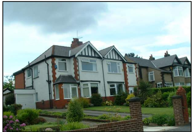
Photograph 106: 26 & 28 Brock Mill Lane (Viewed From Brock Mill Lane)
