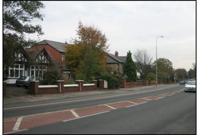
Photograph 8: View south along Wigan Lane, looking towards Broomhey Avenue.
