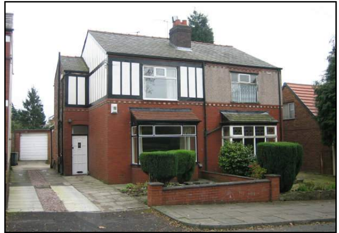
Photograph 25: 10 & 12 Walter Scott Avenue (Viewed From Walter Scott Avenue)
