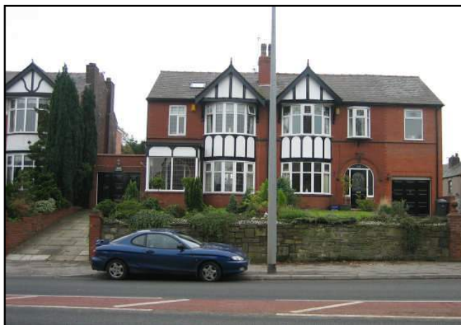
Photograph 22A: 330 & 332 Wigan Lane (Viewed From Wigan Lane)
