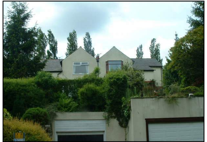
Photograph 103: 14 & 16 Brock Mill Lane (Viewed From Brock Mill Lane)
