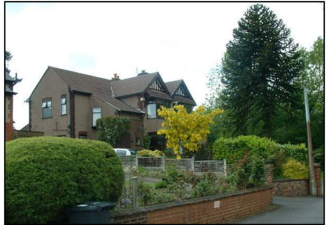
Photograph 108: 34 & 36 Brock Mill Lane (Viewed From Brock Mill Lane)
