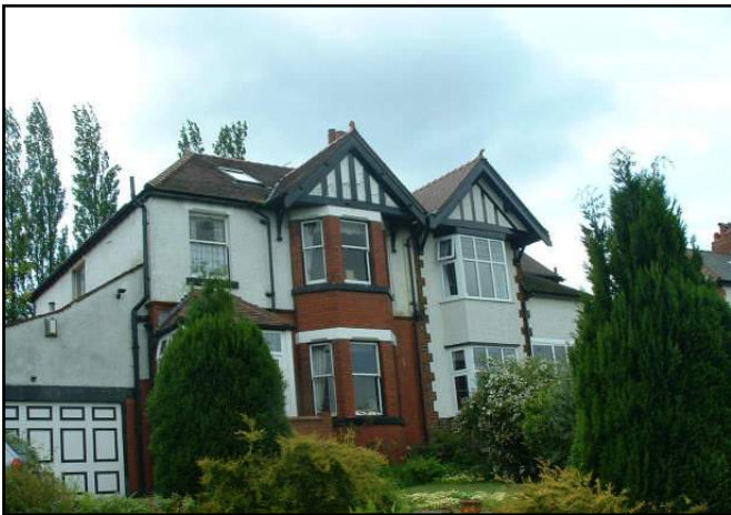
Photograph 105: 22 & 24 Brock Mill Lane (Viewed From Brock Mill Lane)
