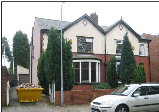
Photograph 23: 2 & 4 Walter Scott (Viewed From Walter Scott Avenue)
