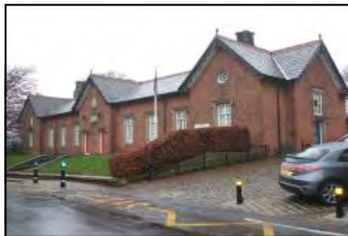
Photograph 14: St David's Church of England School.
