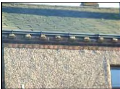
Photograph 15: Example of corbelling details found within the conservation area.
