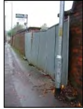
Photograph 41: Metal screening for gap site-unattractive.
