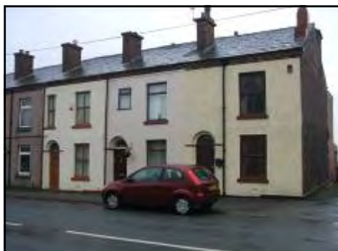
Photograph 16: Examples of various cladding materials within conservation area.
