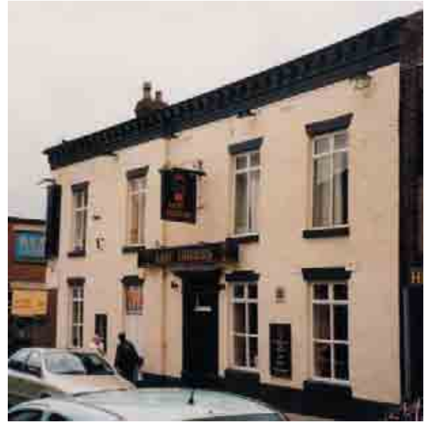
The Last Orders public house retains Doric doorcases and a heavily moulded brick eaves cornice.
