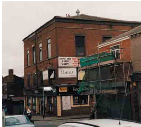
The former Co-op premises (1864) are an important early example of retail development by the co-operative movement.
