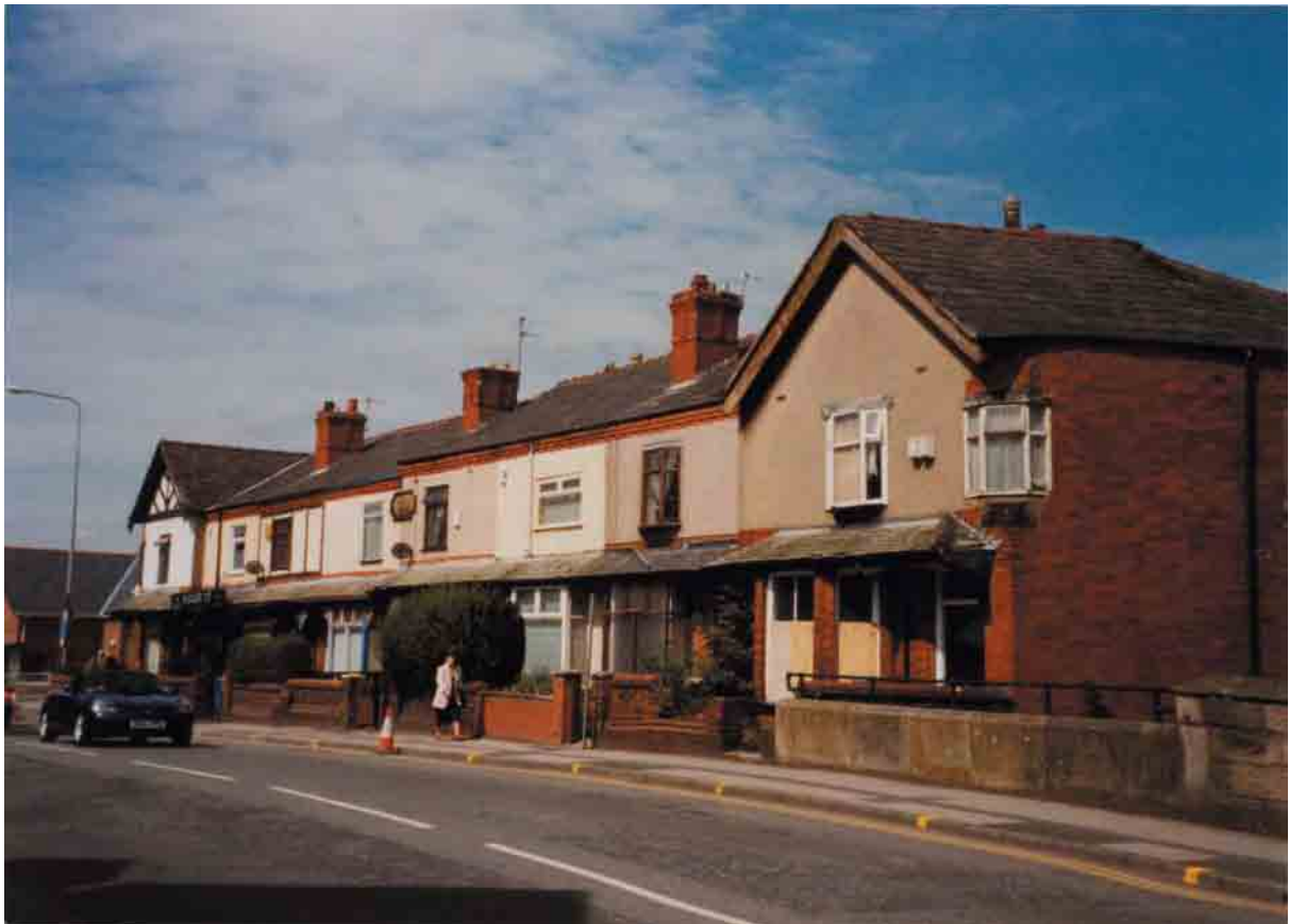
Borsdane Terrace, Atherton Road is carefully composed with attractive detailing which is being eroded by alterations.
