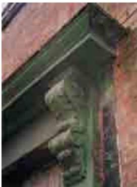
No.22 Bridge Street. A surviving late Victorian shopfront with high quality joinery
