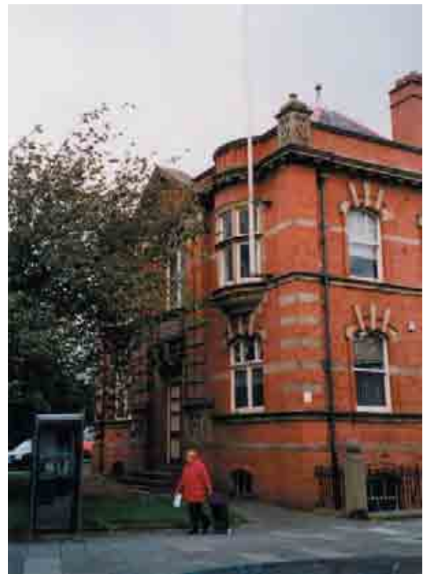
The former offices of Hindley Urban District Council (1903) are an unspoilt example of a civic building in the Queen Anne Revival style.
