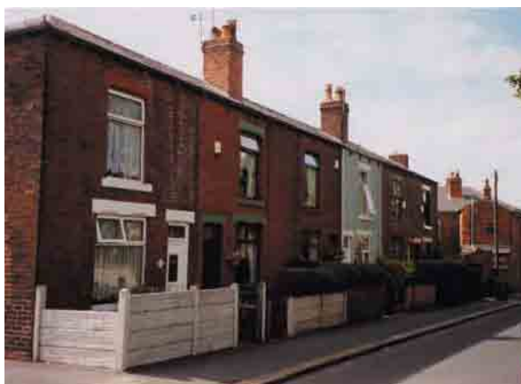
Peter Street. The replacement of timber box sash windows and doors and the removal of mullions from ground floor windows has destroyed the original unity of the terrace. The erection of concrete boundary walling and fences detracts from the streetscape
