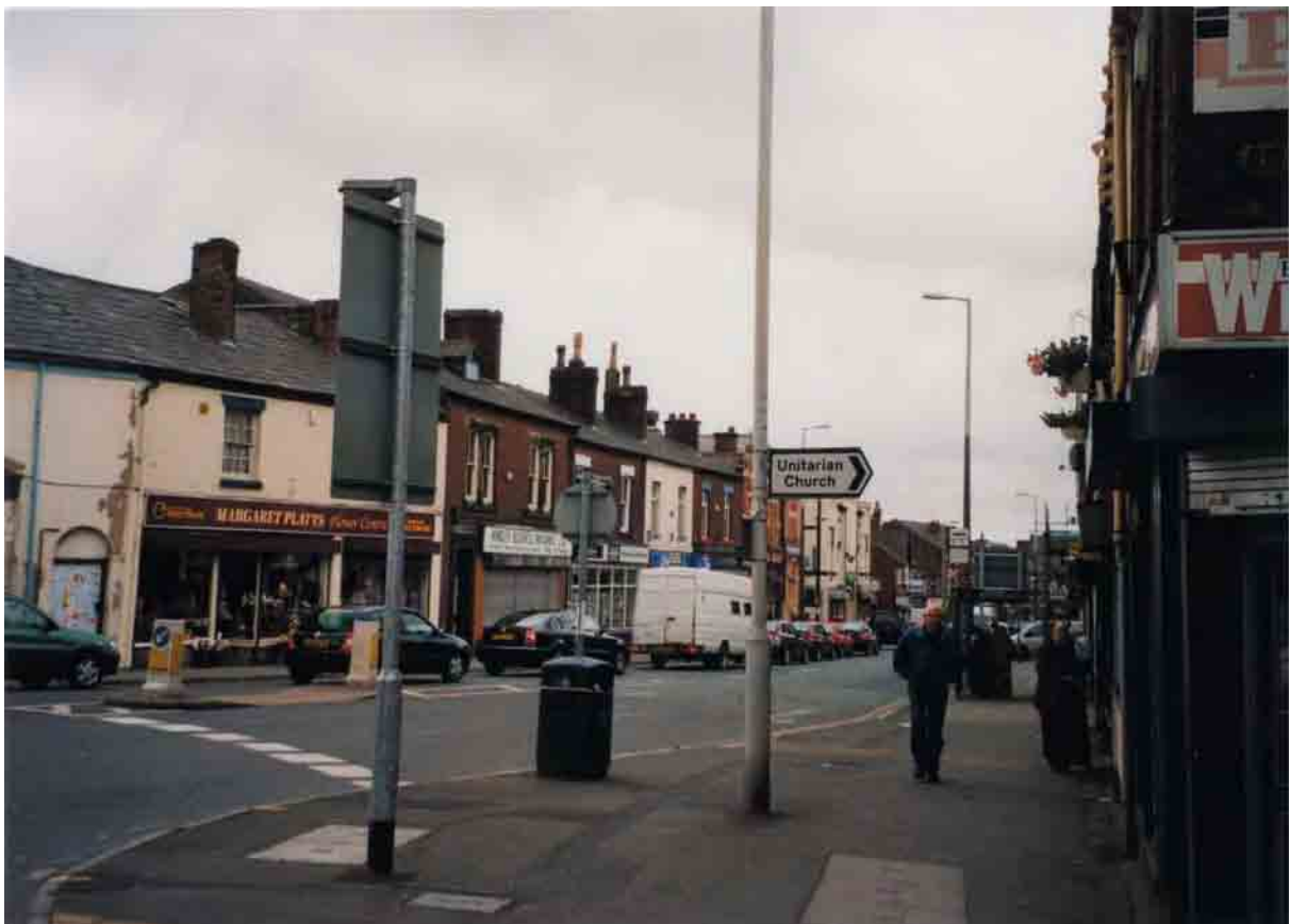
The public realm at the northern end of Market Street is cluttered and unco-ordinated with low quality surface finishes.
