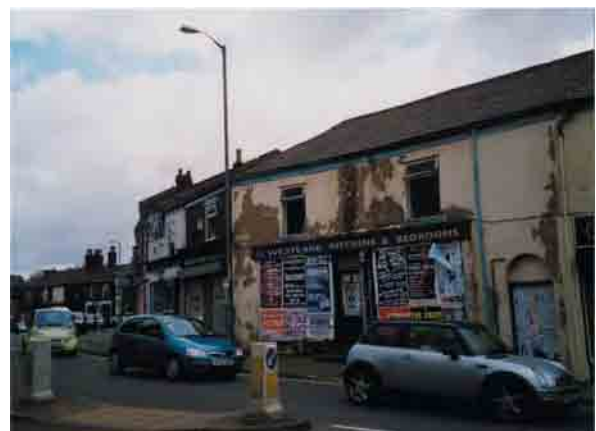
No.21 Market Street ‘AT RISK’.
