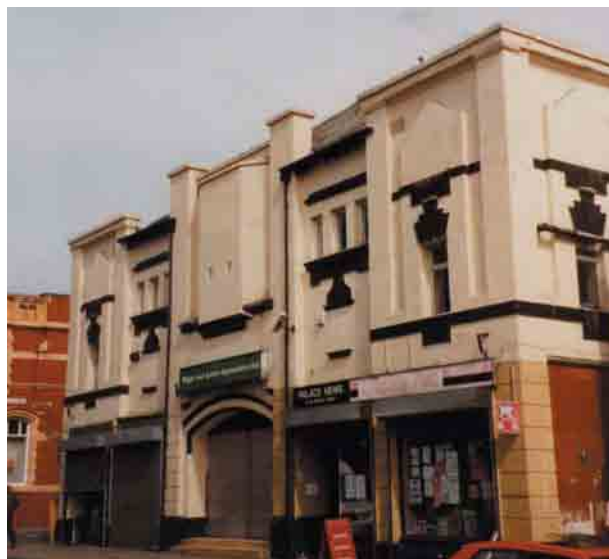
The building today. Whilst unfortunate alterations have robbed the building of some of its impact, these changes are reversible.
