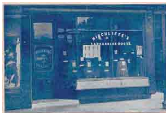
A former traditional shopfront in Market Street (Hinchcliffe’s Lancashire House)
