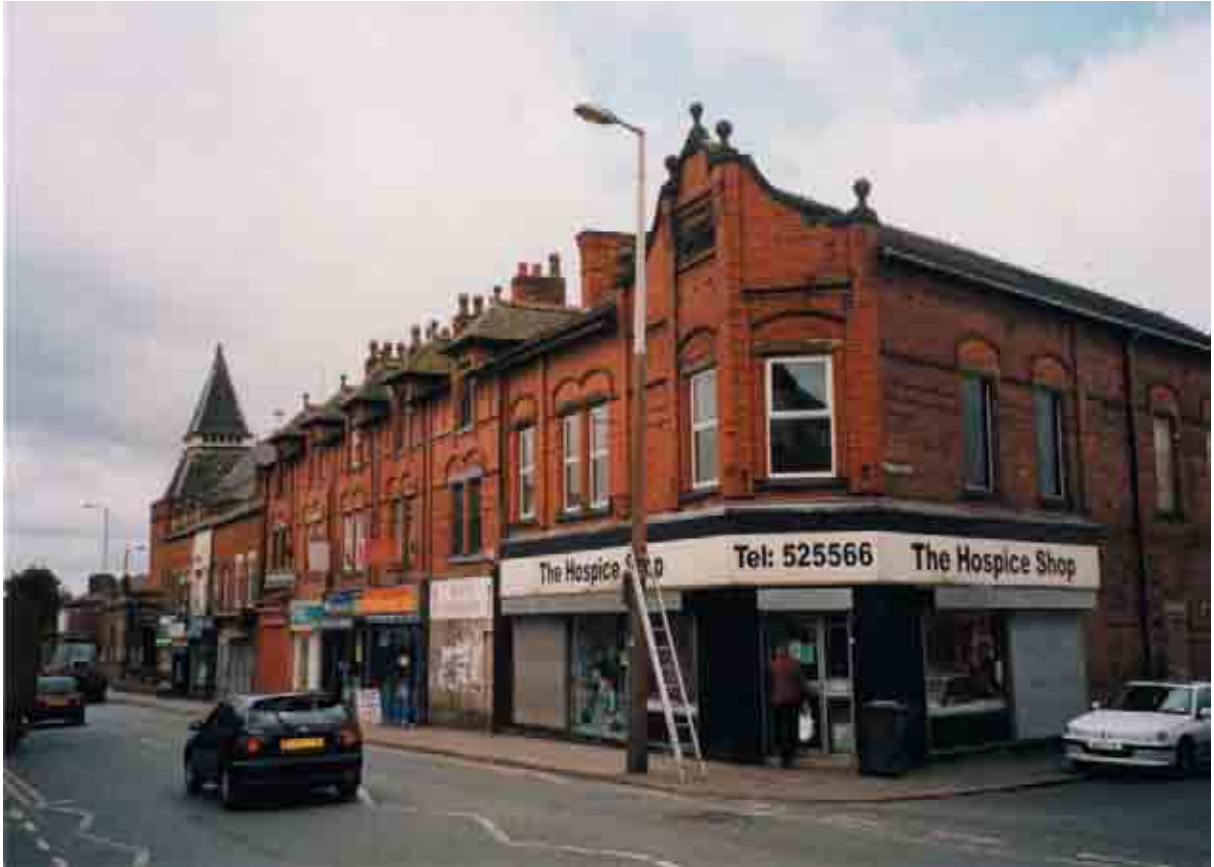
Market Buildings Nos. 78-88 (even) Market Street: A robust parade of late nineteenth century shops marred by replacement shop fronts.
