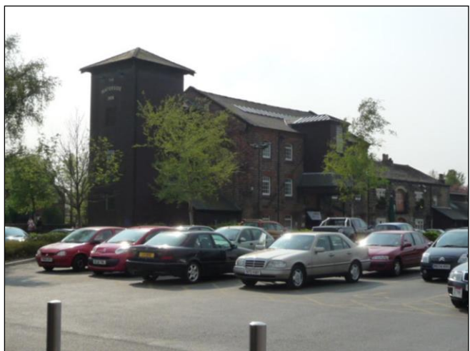
Photo 48: Car Park to rear of Waterside Inn softened by tree planting
