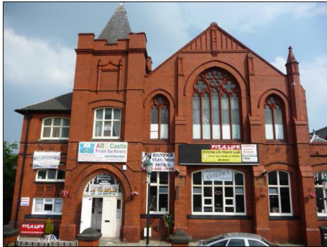
Photo 25: Former King Street Methodist Church School
