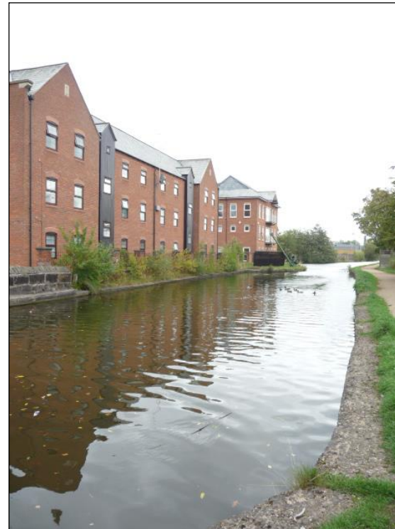
Photo 51: View from Leigh Bridge eastwards
