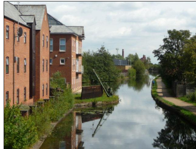
Photo 19: New apartments and office block on the north side of the Bridgewater Canal
