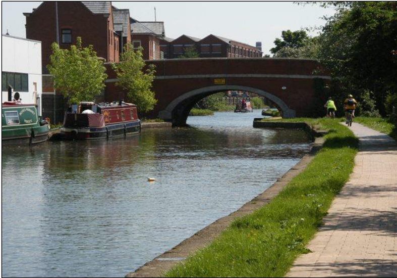
Below: photo 33: Leigh Bridge
