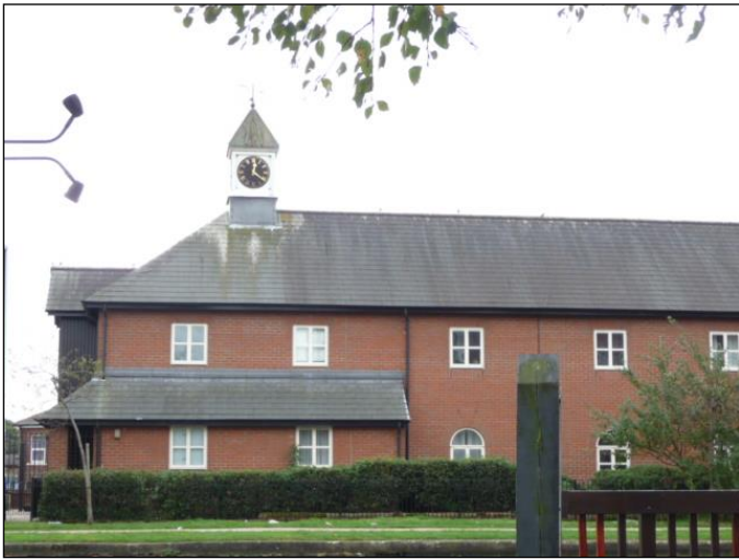
Photo 13: Ropewalk apartments fronting the south bank of the Bridgewater Canal to the west of Leigh Bridge
