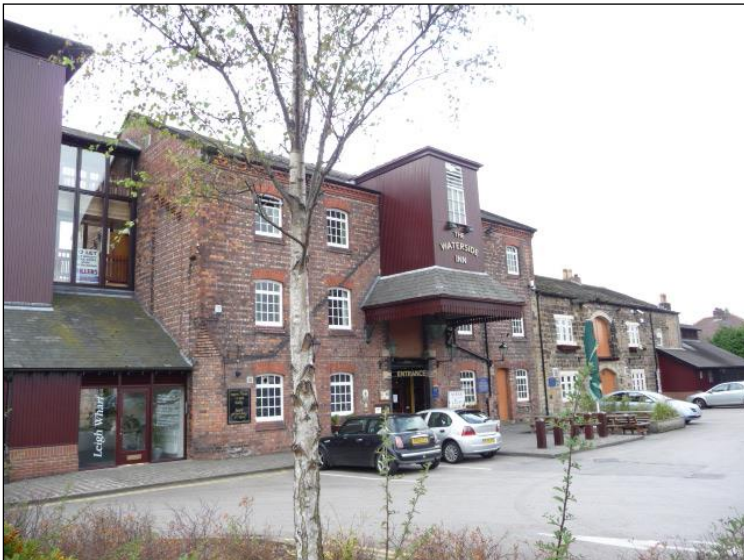
Photo 29: Former Canal Warehouse (front elevation)
