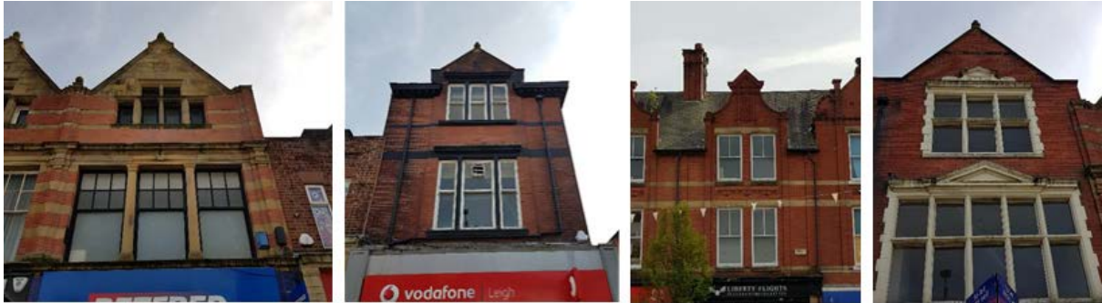
Picture 6.14 Details at upper floors such as stone dressings, timber windows and ornate terracotta gables with finials.
