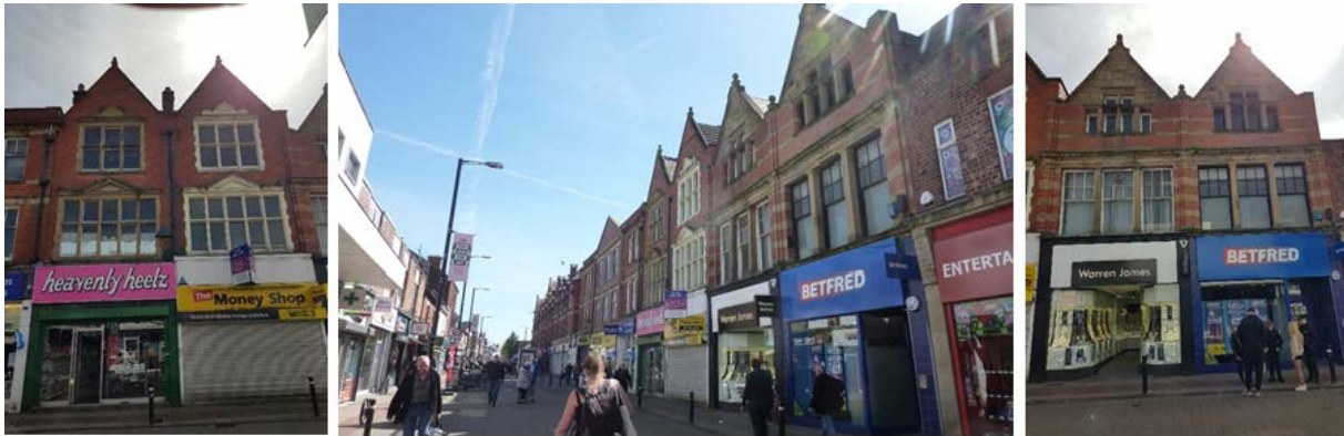
Picture 6.3 Prestwich designed buildings characterise the north side of the street, notable for their pressed red-brick and stone details as well as varied gables.
