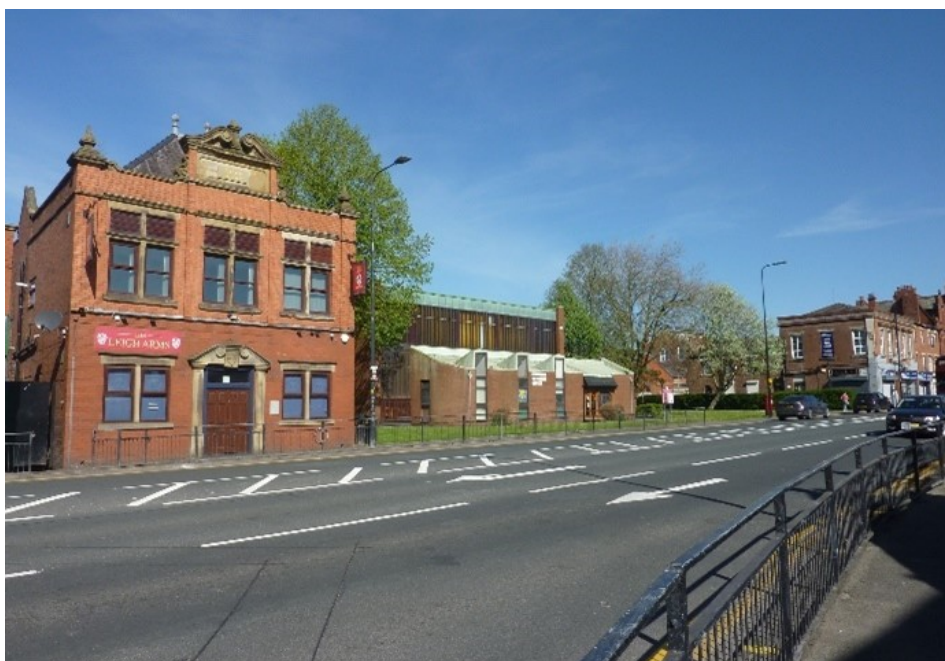
Picture 4.13 Strong building lines broken by poor infill development
