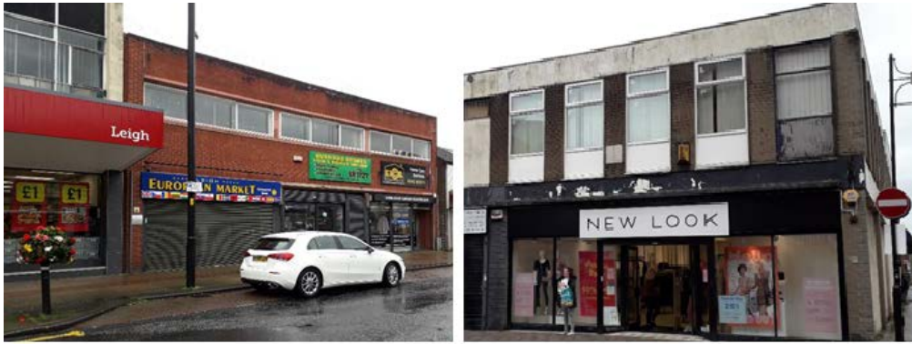
Picture 6.17 Inappropriate infill with scale, style, materials and fenestration are not positive contributors to the conservation area.
