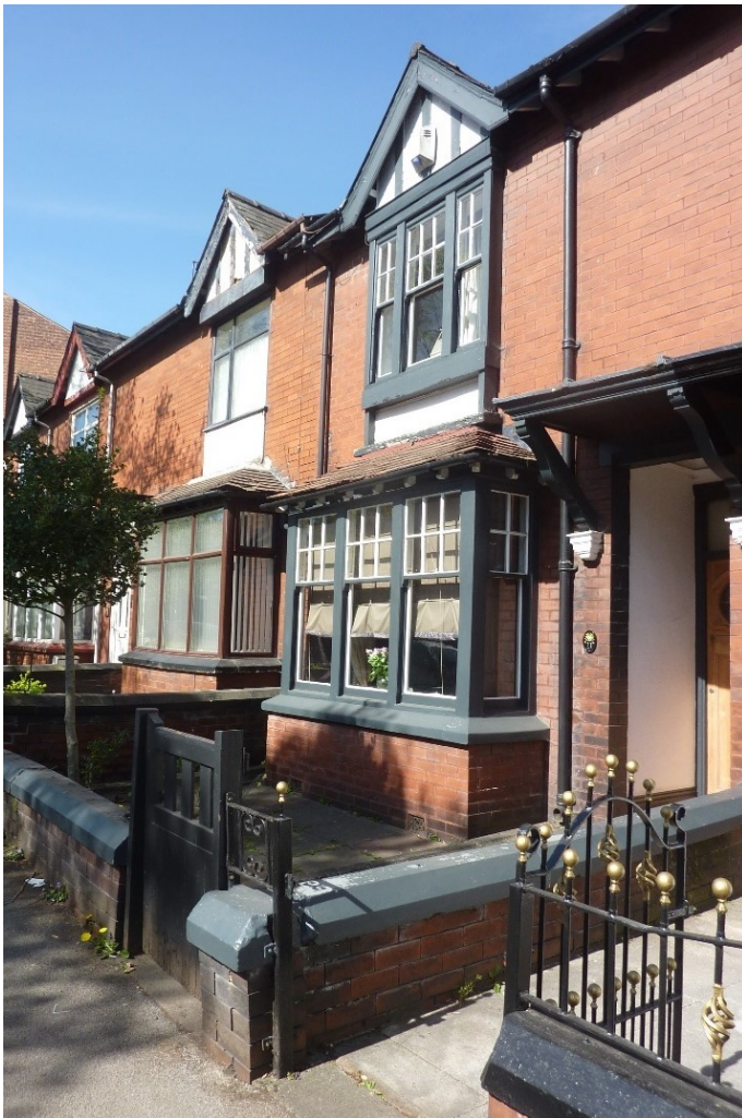
Picture 4.10 Timber details on The Avenue
