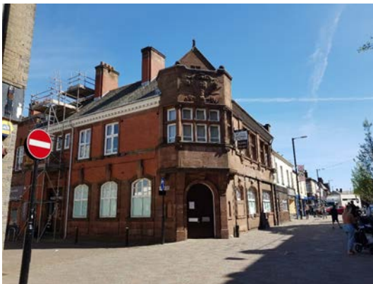
Picture 6.4 Prominent features on street corners break up the geometrical layout.
