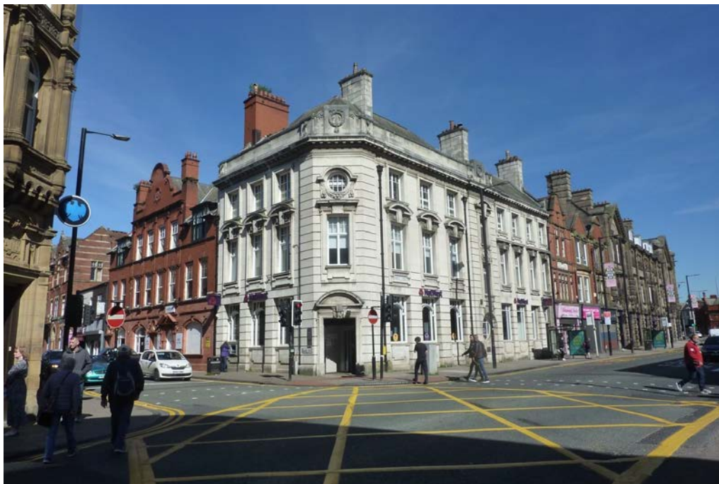
Picture 2.1 Looking along Railway Road and Market Street there are eclectic styles of grand Victorian architecture.
