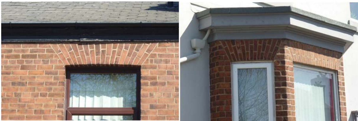
Picture 5.9 Gauged brick window heads with large splays are a feature of this area..
