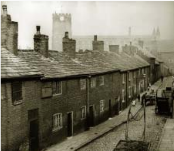
Back Salford c.1905. Note the window frames and sandstone roofs.
