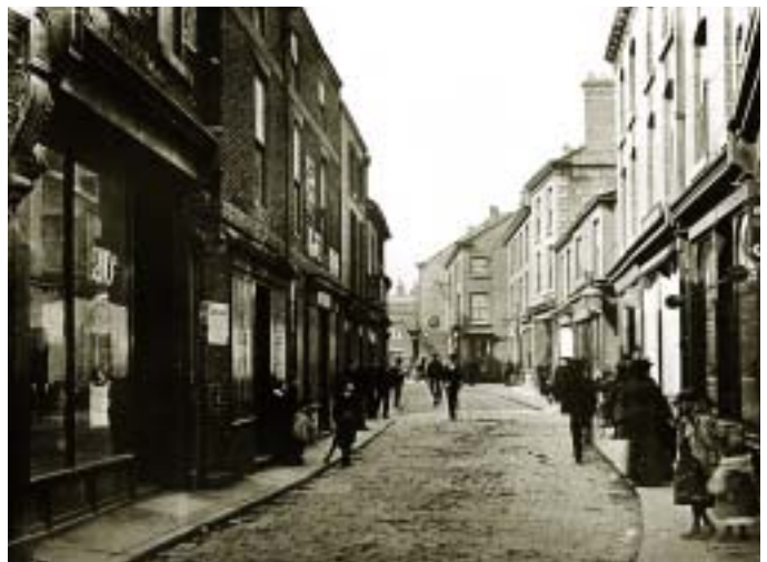
Market Street, looking north, prior to widening.
