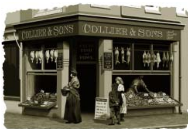
No. 40 Railway Road with its wide sash display windows, typical of fresh food shops, e.g. butchers. (See page 39).
