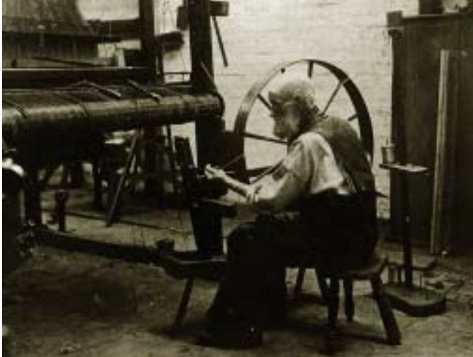
Silk hand-loom weaver operating a winding machine prior to weaving on the loom to left.
