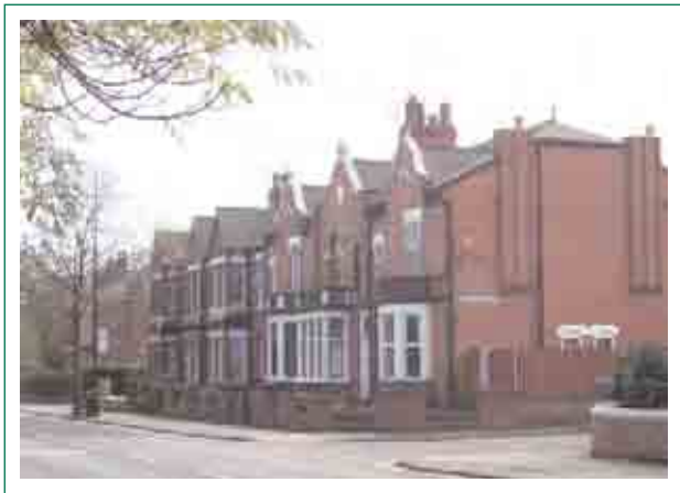
Nos 5-10 Park Road.
