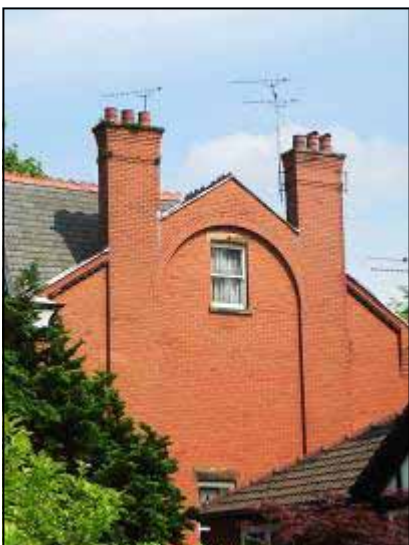
Photograph 11(left): Red brick which is common throughout the conservation area.
