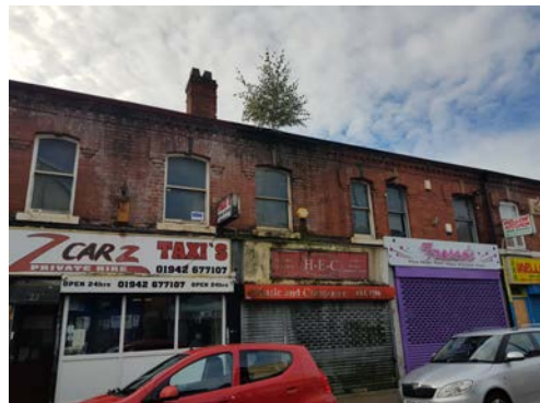
Picture 3.16 Original sash windows largely survive on this terrace..
