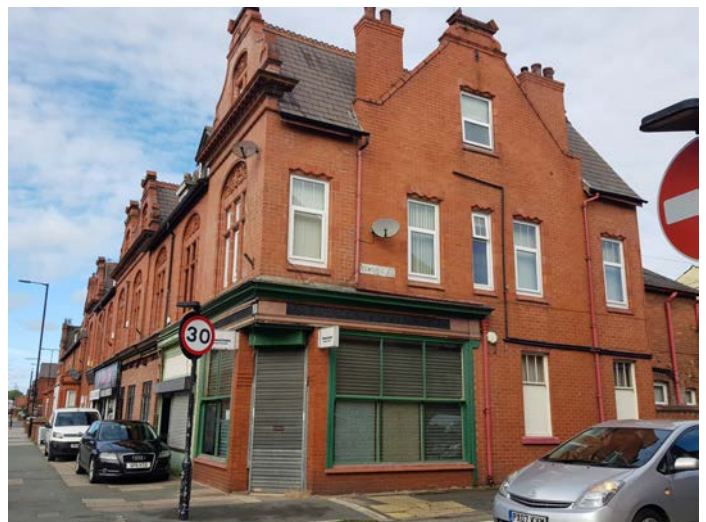
Picture 3.18 Notice the very large sliding-sash windows. A rare survival.
