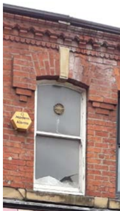
Picture 2.3 Decorative brick window heads and a surviving sliding-sash window.
