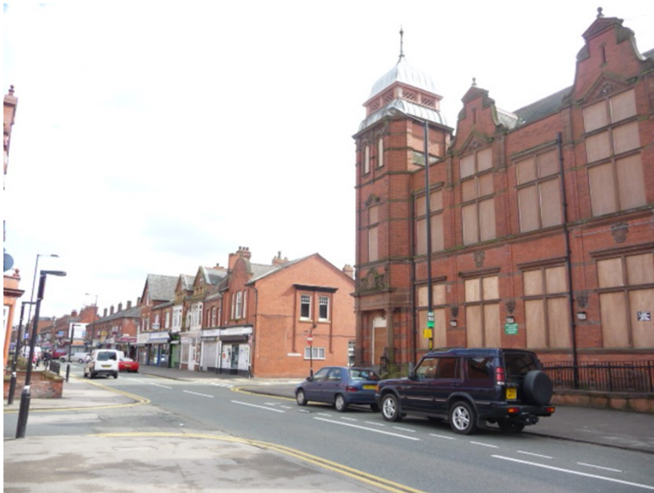
Picture 3.5 The former College building is substantially taller than other buildings in the conservation area.
