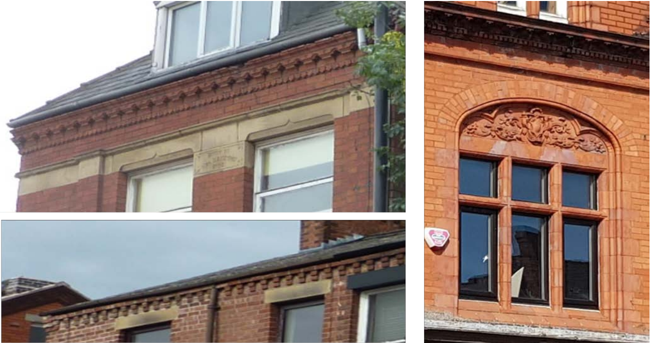
Picture 2.1 Decorative stone and terracotta are a feature found on cornice bands and windows.
