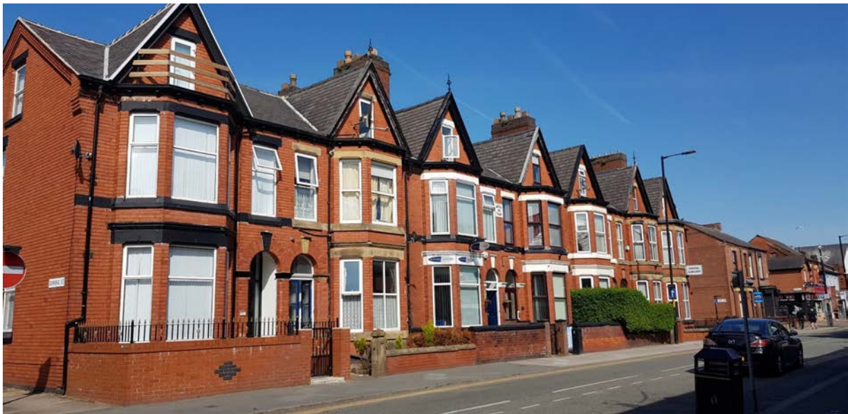
Picture 3.9 The terrace comprises sizeable two storey houses, with attic floors lit by a single window within steep gables.
