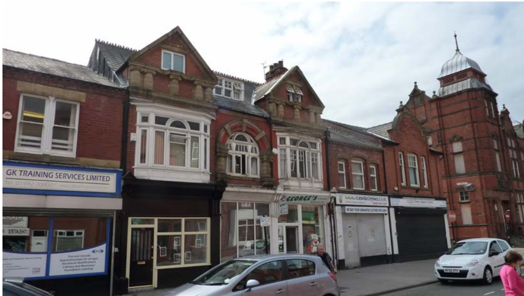
Picture 3.14 The fine architectural details of the former Leigh Friendly Co-Operative Society Headquarters are the highlight of this terrace.
