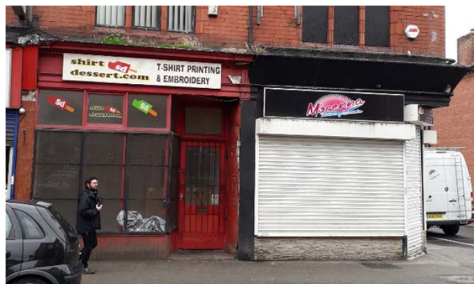
Picture 2.6 Recessed shop doorways and original windows can be seen behind modern security grills - roller shutters hide these features
