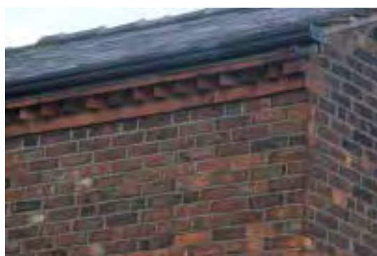
In many cases the differing eaves detailing could have been the individual builders mark and provide a simple variation and individuality.
