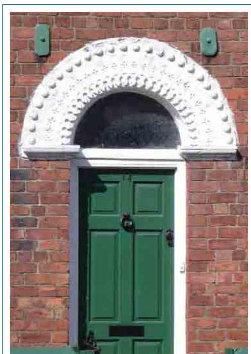
Doorway no.14 Cross Street
