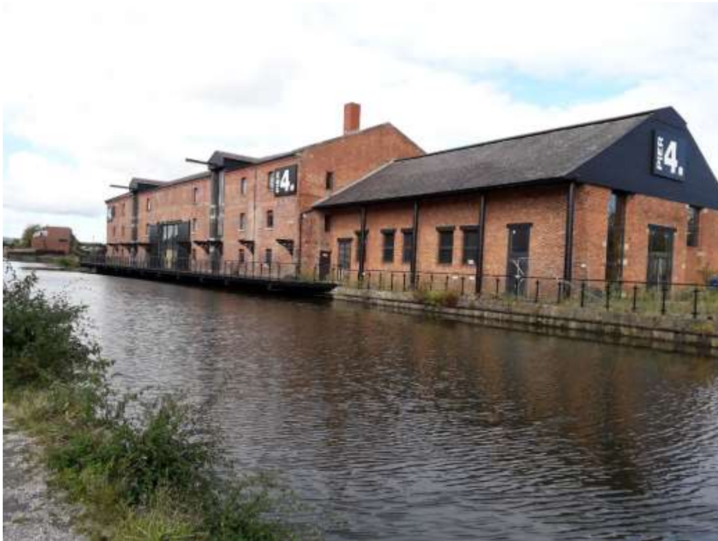
Picture 1.7 – Pier 4 from the canal
