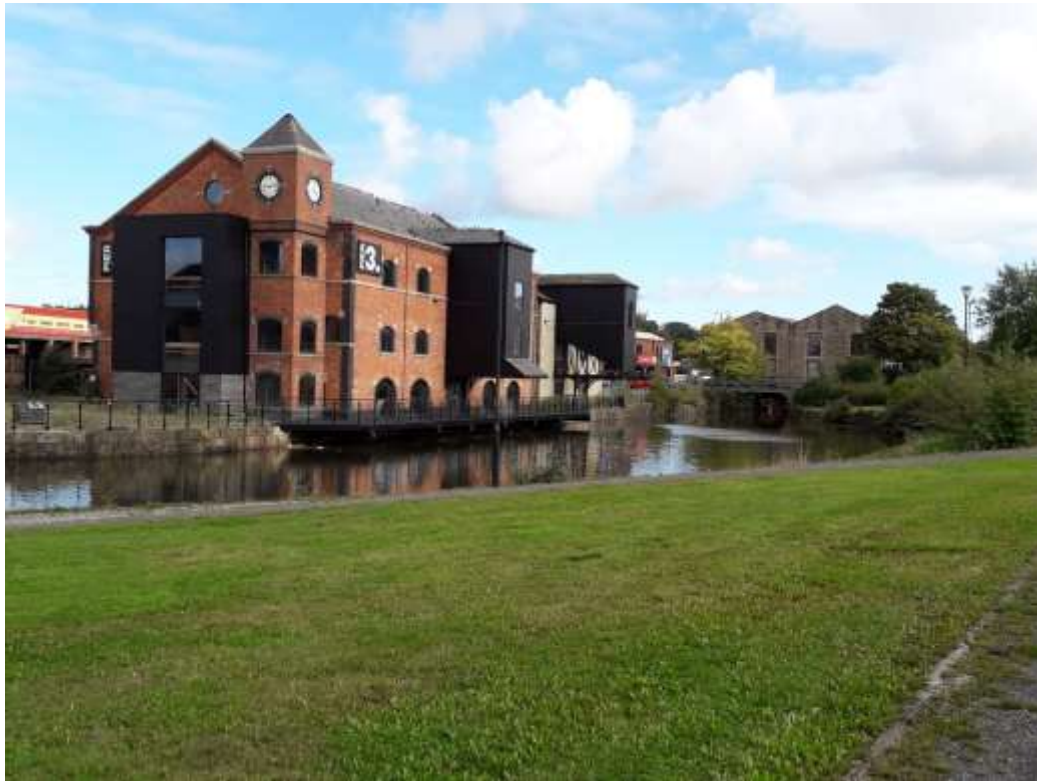
Picture 1.6 – Pier 3 & Terminal Warehouse from the canal
