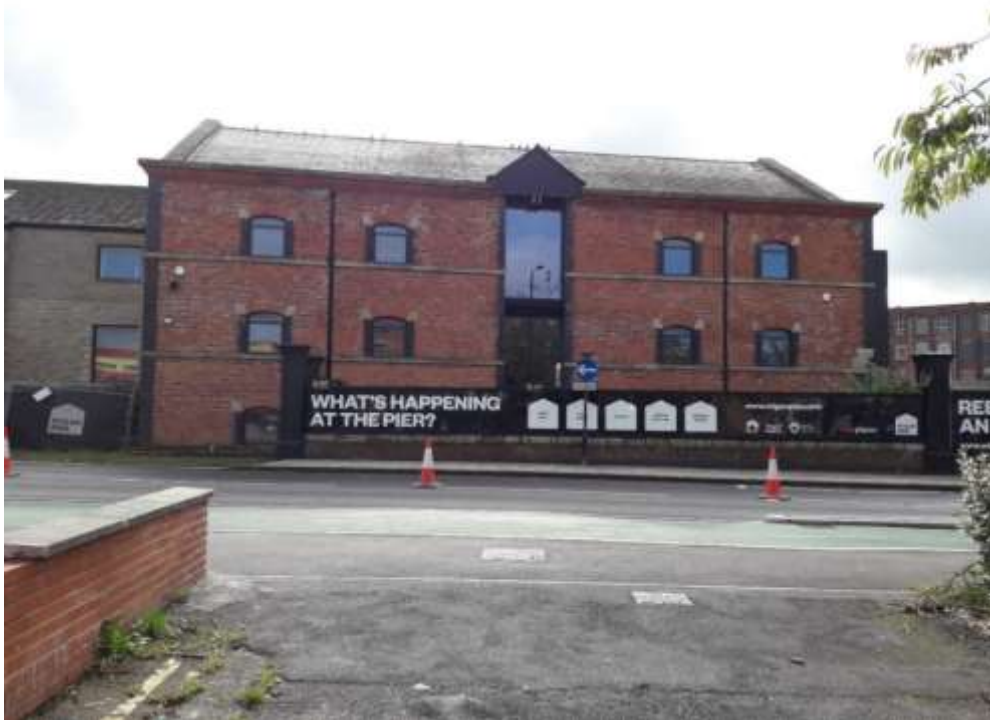
Picture 1.4 – Pier 3 (formerly The Orwell Public House), from Wallgate
