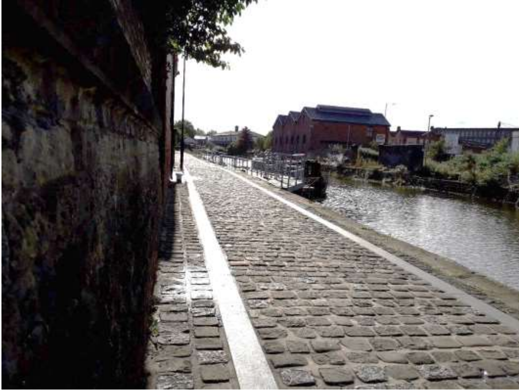
Picture 1.9 – Leeds - Liverpool Canal, from adjacent Pottery Bridge
