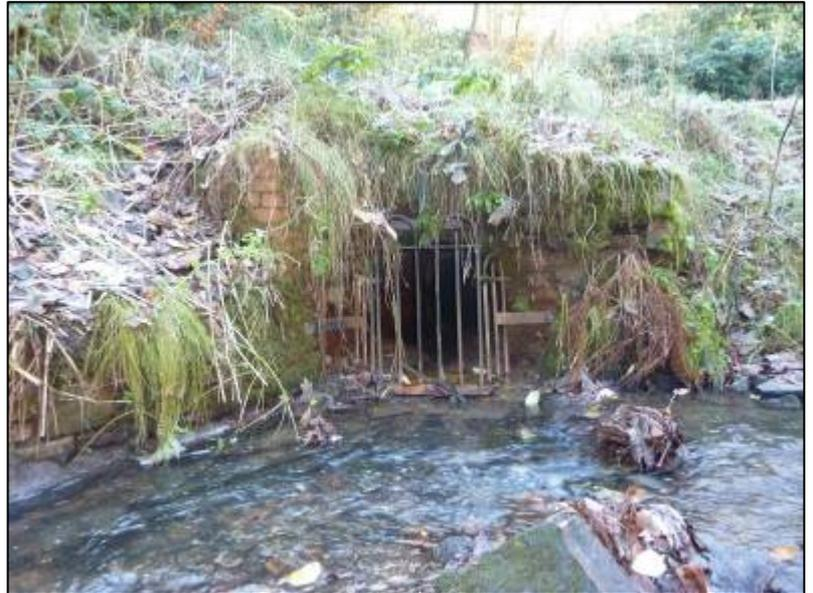
The entrance consists of two brick pillars supporting a large concrete slab over the brick archway of the drain itself. An iron grille has also been fitted across the opening. The entrance is in reasonable condition; some of the bricks on the right-hand side of the arch have slightly deteriorated but are stable. Vegetation has grown over the brick pillars and concrete slab.
