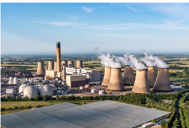
Coal-fired power station
